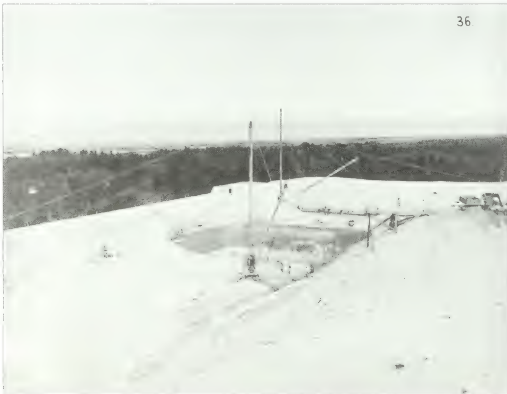
Figure 2.21. Placing sand around the northwest mortar pit, the Mortar Battery, 1893. Vertical concrete walls rose up from each mortar platform and met a concrete blast slope that tapered to a wider opening. The vertical walls and blast slope held back the Mortar Battery's engineered earthwork (Lee and Laham, Historic Structure Report ).
